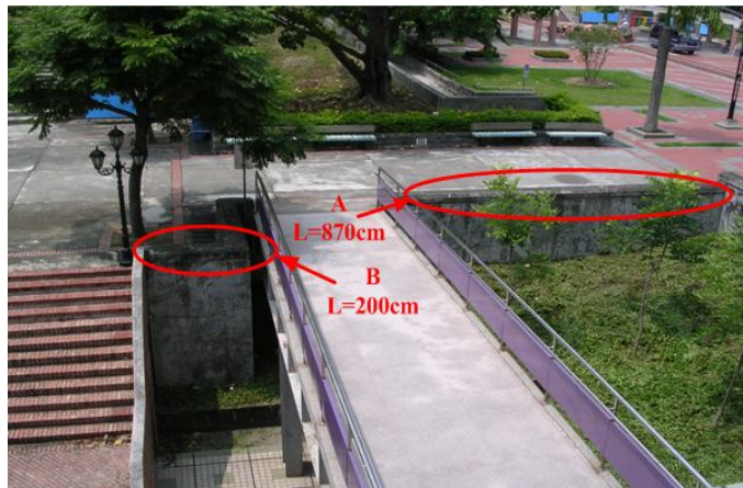
Figure 13. Photograph of the earth retaining walls tested
