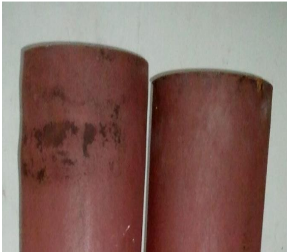
(a) local buckling at the ends
