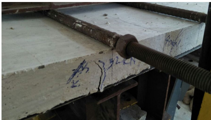
Fig. 19. Crack at mid-span of FET2SS1 composite slab
