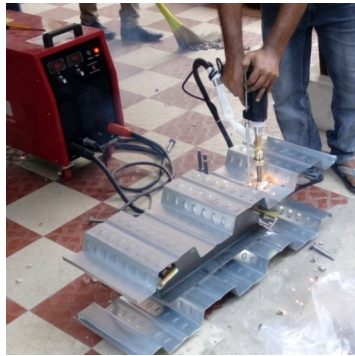
Fig. 5. Gun welding in progress
