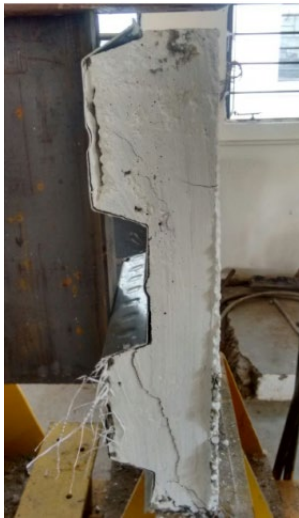
Fig. 24. Crack pattern on the sides of 'PET1'
