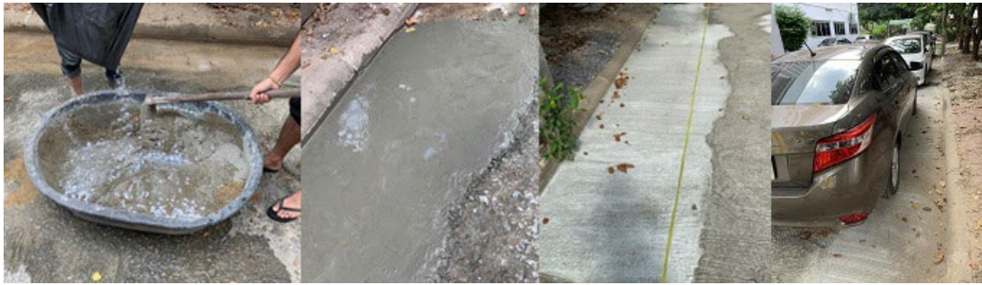
Fig. 7. The resurface of the pavement around the roads inside Chandrakasem Rajabhat University by ECPA
